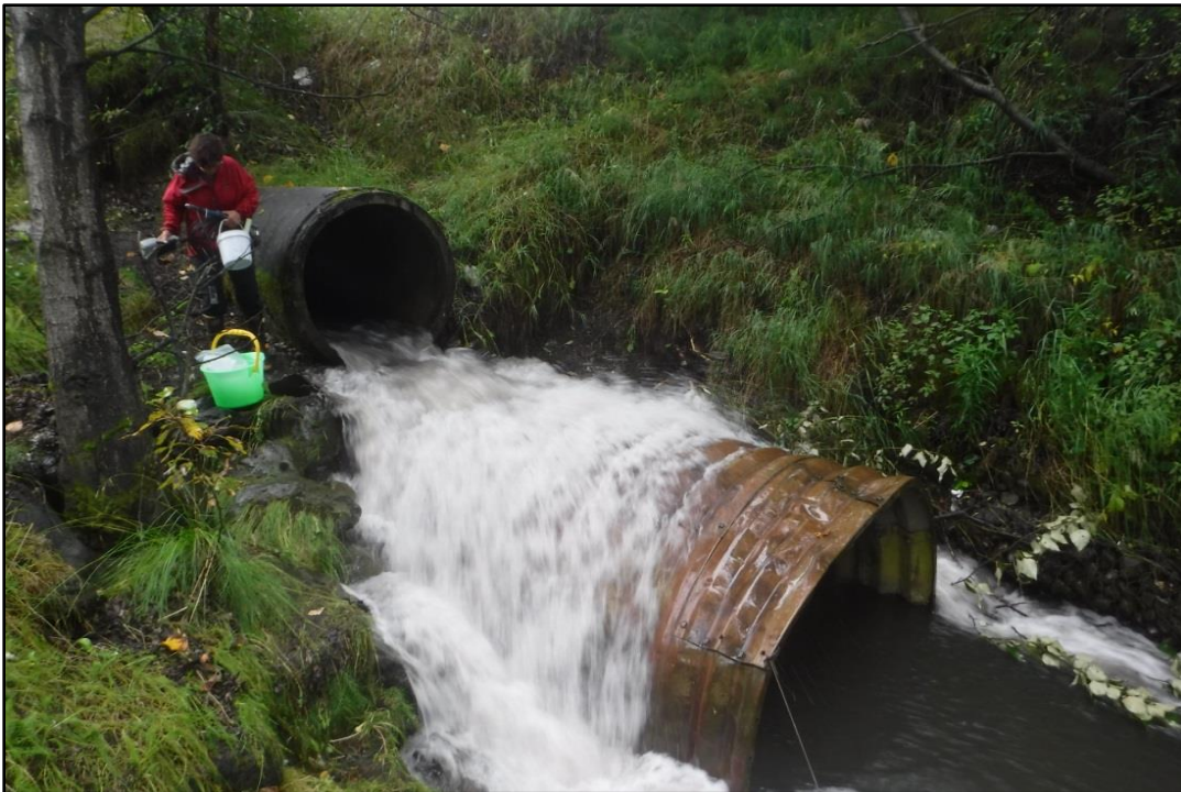
Photograph 8. Outfall SWM08 (86-1), New Seward Highway at Chester Creek.
