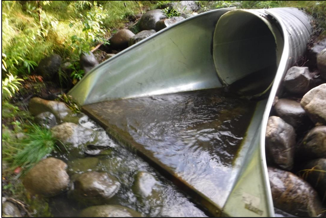
Photograph 3. Outfall SWM03 (1224-1), Fairweather Loop off Sylvan Drive.
