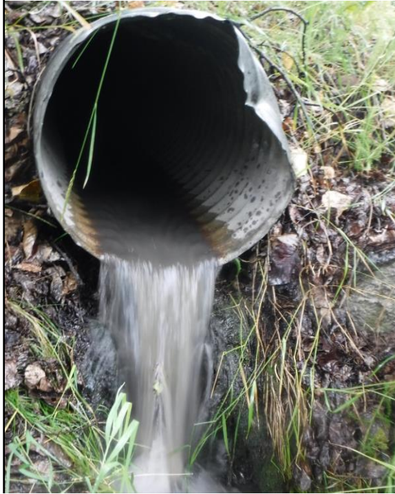
Photograph 7. Outfall SWM07 (484-1), New Seward Highway at Chester Creek.
