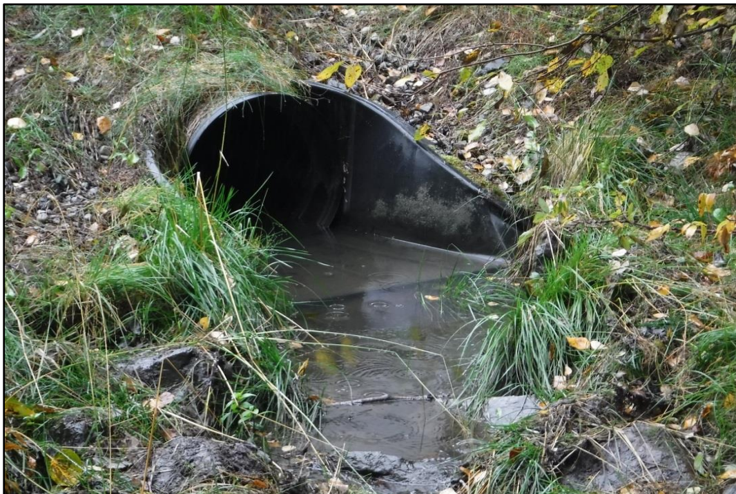
Photograph 4. Outfall SWM04 (1224-2), Fairweather Loop off Sylvan Drive.
