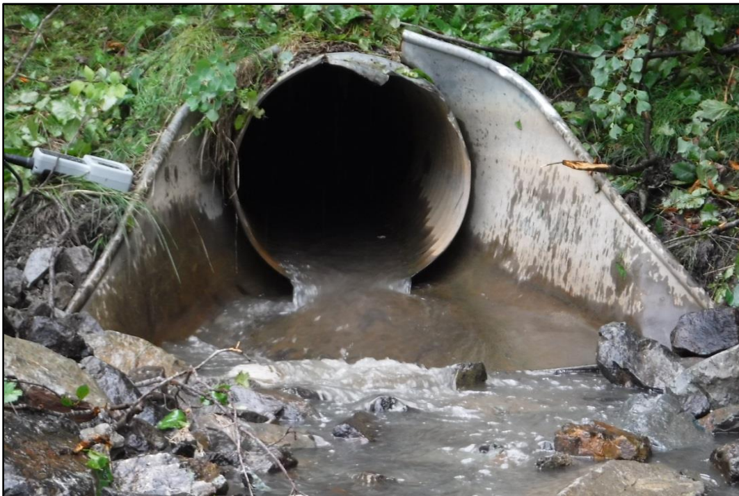
Photograph 2. Outfall SWM12 (1454-1), Lynwood Retention Basin.
