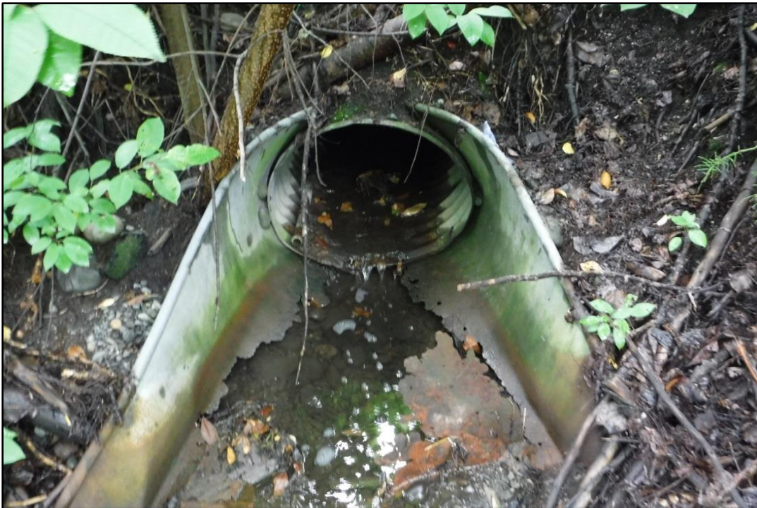
Photograph 6. Outfall SWM06 (314-22), Maplewood Street off of Northern Lights Boulevard.
