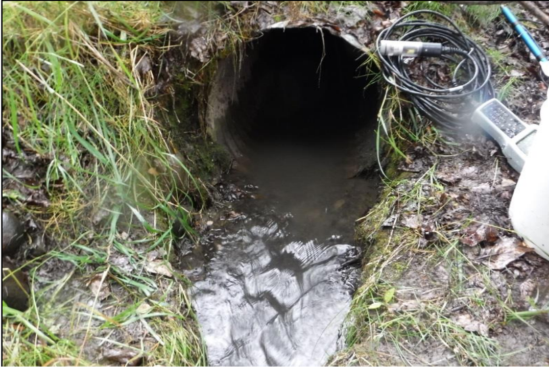
Photograph 9. Outfall SWM09 (499-1), Anchorage Football Stadium & Ben Boeke Ice Arena.
