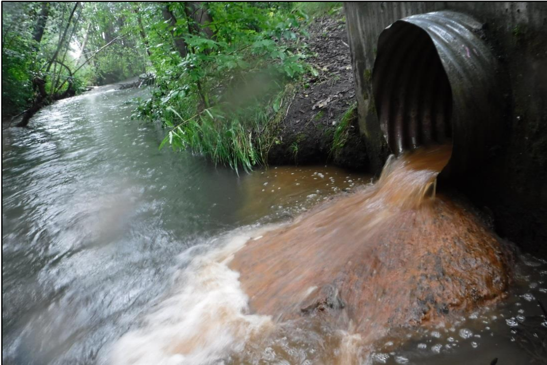
Photograph 10. Outfall SWM10 (525-2), Eagle Street at Chester Creek.
